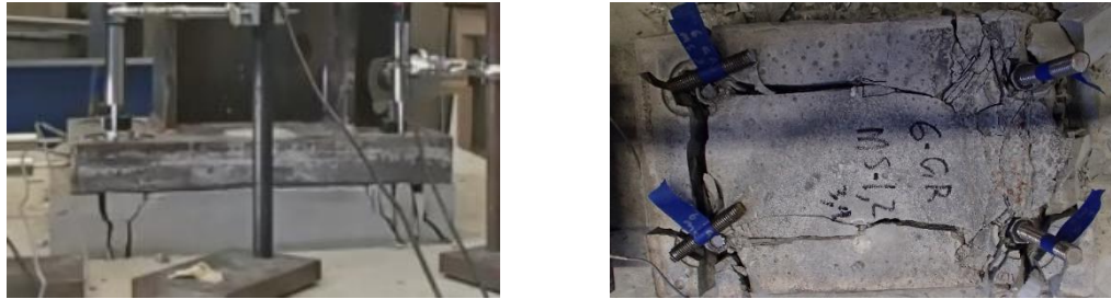
Figure 4. Cracking behavior of grout pads under shear and moment loading: profile view (left) and plan view (right).
